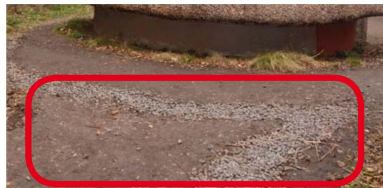
*Within the Village a number of drainage gullies had been cut and filled with aggregate. These produced an uneven surface. A short term recommendation was made to change this aggregate to a finer-grade.*
