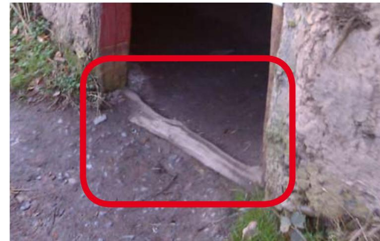
*The low doors and high thresholds into the roundhouses also presented a barrier to access. In addition, disking of the ground surface in front of the door also lead to puddling which exacerbated the trip hazard. These barriers meant that some disabled visitors had difficulty accessing the interpretation within the building, and no alternative was provided.*
